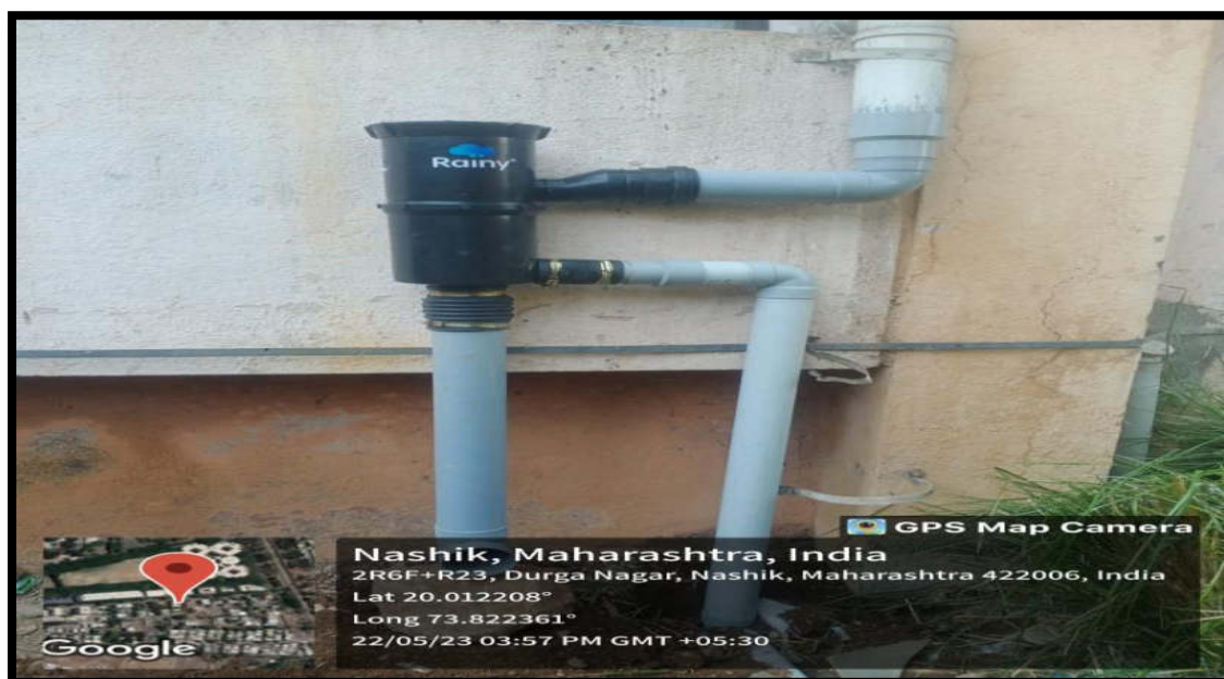
Rain water harvesting facility
